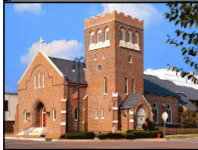
Top to bottom - Saint Luke's during the tornado, during construction, and completed.
